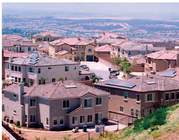
Shea Homes located its two high-performance developments in the Scripps Highlands area of San Diego County.
